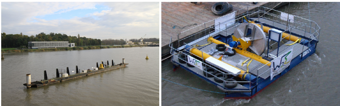
Figure 1: Experimental pontoon installed in the tidal estuary (Sea Scheldt, west of Antwerp) for tidal turbine tests in real conditions (left panel). A vertical axis tidal turbine of the Dutch company "Water2Energy" mounted on a surface floating platform and installed at a side of the pontoon (right panel).
